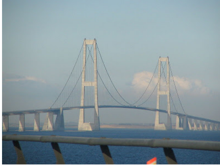
Figura 30 – Ponte Great Belt Bridge
