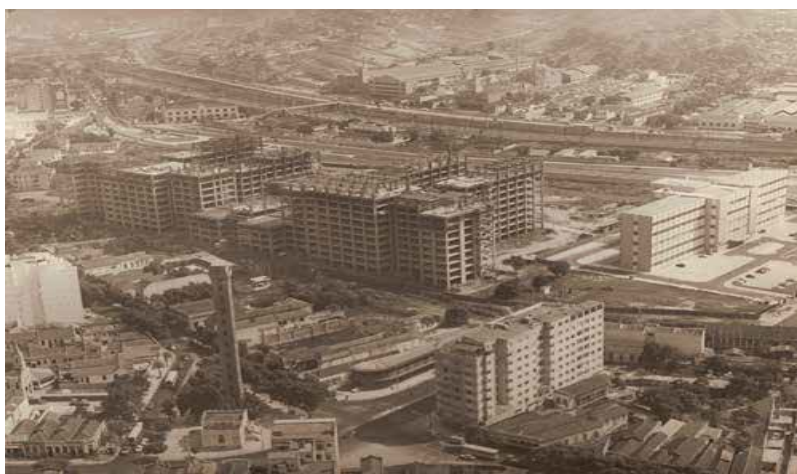
Figura 1 - Campus Maracanã durante as obras.dc. 1970, [s/autor]
