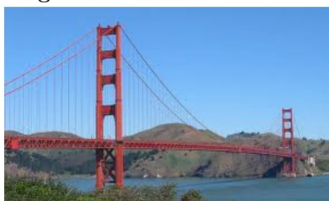
Figura 6.3: Ponte Golden Gate
